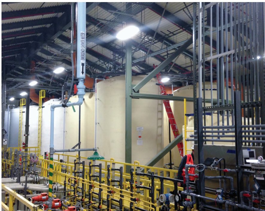
Sulfuric acid storage tanks at a water treatment plant.
