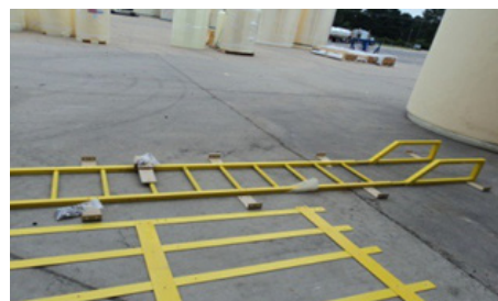
Photo showing location for cage attachment brackets to ladder railing (8 total). Heads of bolts are on climbers' side of ladder.
