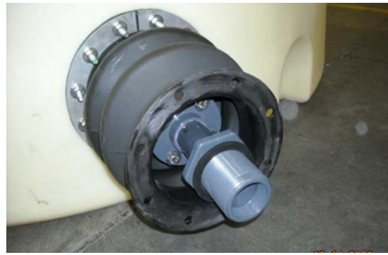
INSTALL BELLOWS HOUSING AND 8" SPLIT RING USING THE PROVIDED HARDWARE. NOTE: AFTER ASSEMBLY IS GLUED REMOVE GASKET FROM BHF AND CHECK WITH A STRAIGHT EDGE. TO ENSURE ALL SEALING SURFACES ARE ON THE SAME PLANE.
