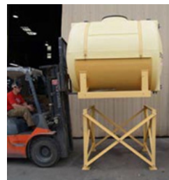
Place Tank on Stand
