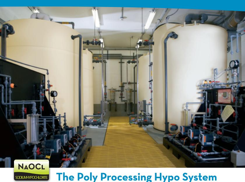
Poly Processing's Sodium Hypochlorite Storage Systems are specifically designed for containment of this challenging chemical. By using carbon black, white or gray compound XLPE resin, **UV degradation of the chemical can be dramatically reduced**. Mastic coatings and insulation are other ways to reduce UV's effect on the chemical.
