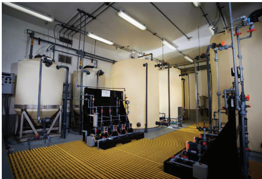
Crosslinked polyethylene tanks are NSF/ANSI/CAN 61 certified for use with a number of chemicals.
